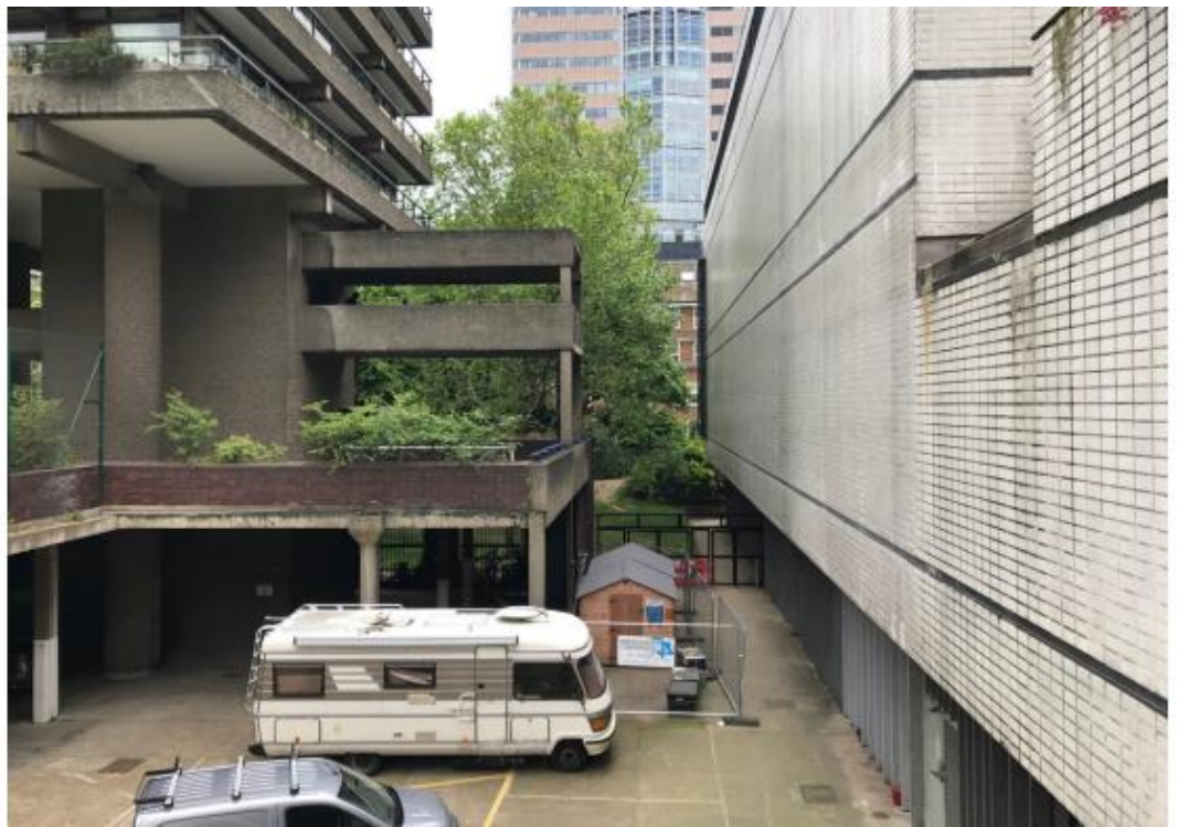
Mountjoy Close existing, car park and northern boundary to Barbican Estate and MoL with Barber Surgeons Garden in the distance
